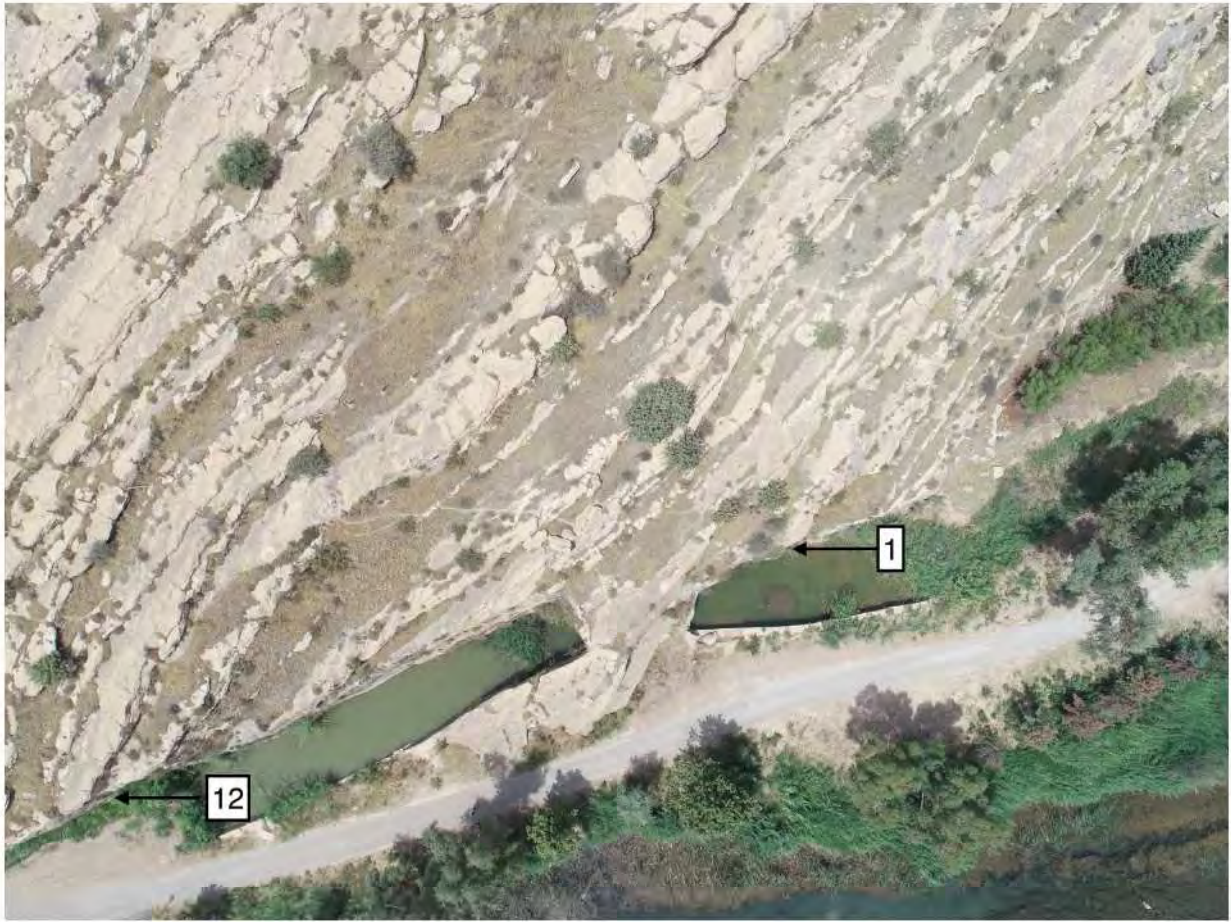
Figure 9: UAV view of the canal and tunnel through the rock spur and location of the twelfth and first rock stelas.
