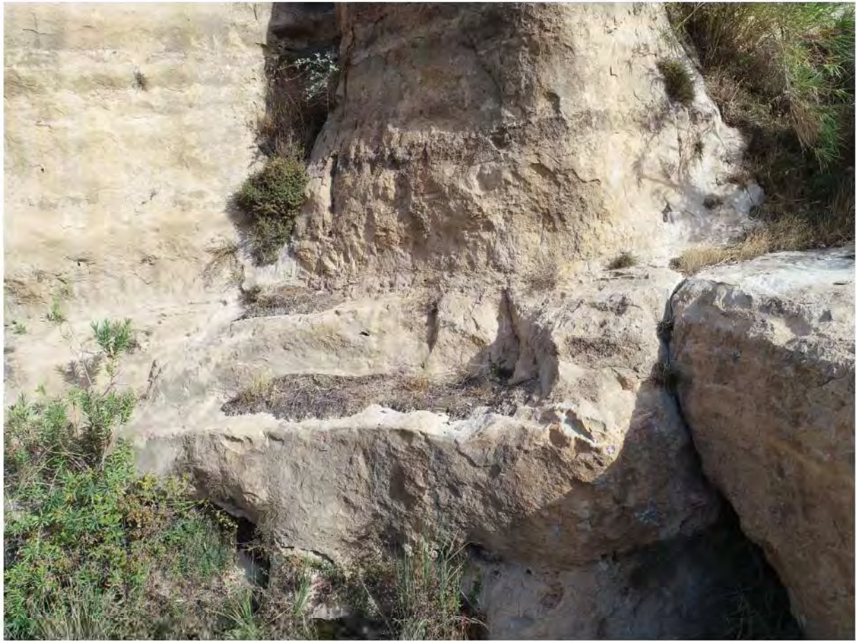
Figure 14: UAV view of Panel C.
