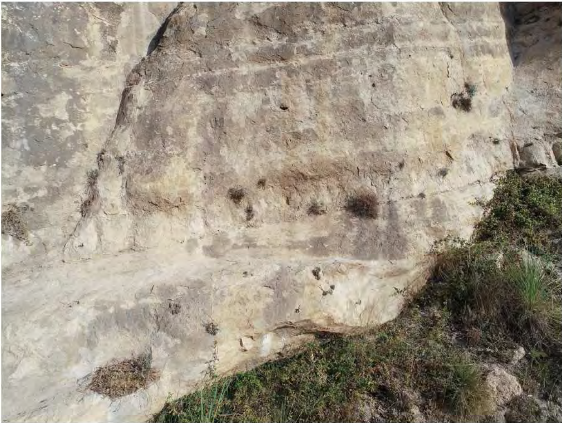
Figure 13: UAV view of Panel B.
