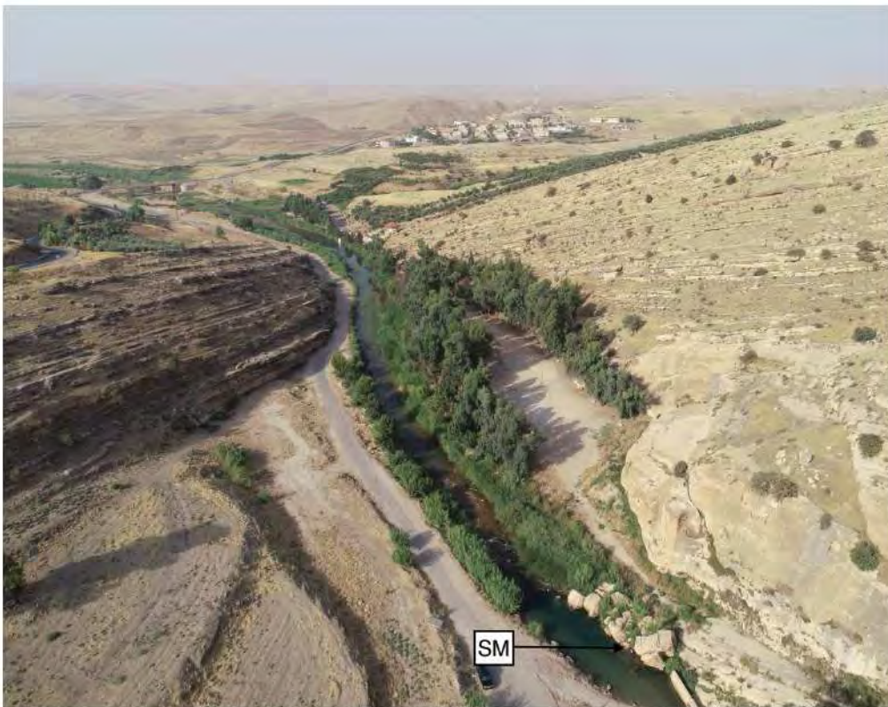
Figure 4: UAV view of the Khinis quarry from the NE with inclined limestone beds on both riverbanks (image top) and horizontal beds to the north of the Sculptured Monolith at the canal gate (SM) (image bottom).
