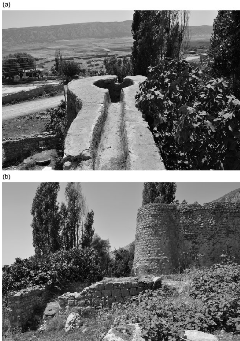
Fig. 15 a) Channel bringing water to the gristmill drop-tower (note the opening in the cylindrical holding-tank); b) channel, drop-tower and millhouse, Yekmala (site 315). © LoNAP
