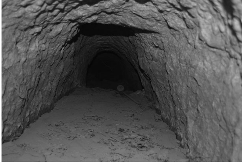
Fig. 14 View of the Bandawai water tunnel (note the river sediments deposited inside). © LoNAP
